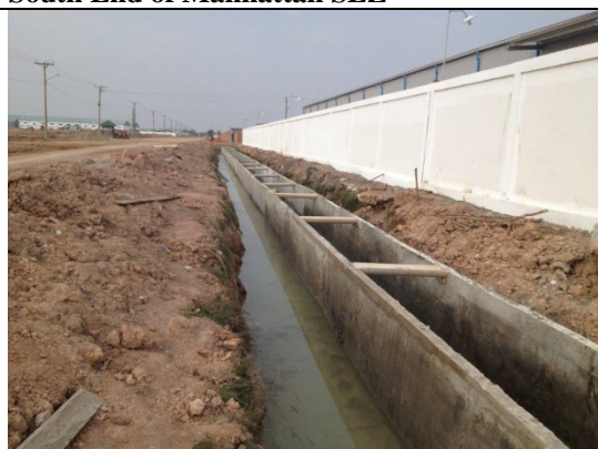
Photo 7.3 : Rain Water U-channel has been installed (Manhattan SEZ)
