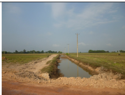
Photo 7.7 : Small Ditch to be Maintained at the North Side of Tai Seng Bavet SEZ Sub for Constant Discharge
