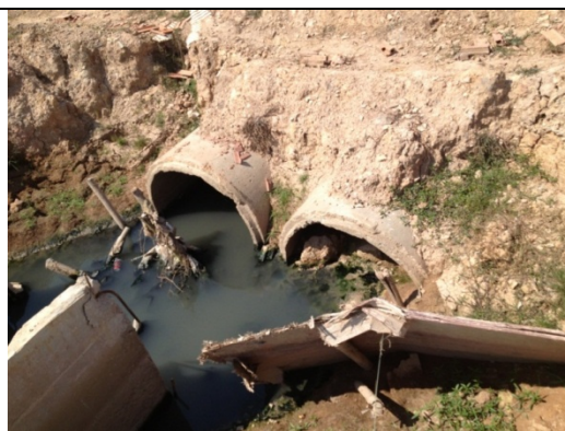
Photo 7.2 : Waste Water Pipe and Rain Water Pipe, Separate System (Manhattan SEZ)
