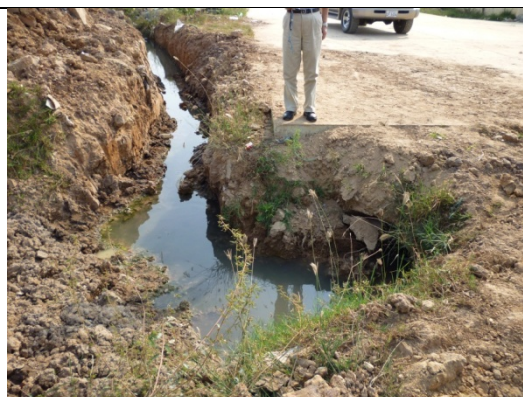
Photo 7.5: Effluent Condition, One Pipe for Waste Water and Rain Water (Tai Seng Bavet SEZ Sub)
