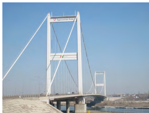
Irtys River Suspension Bridge
