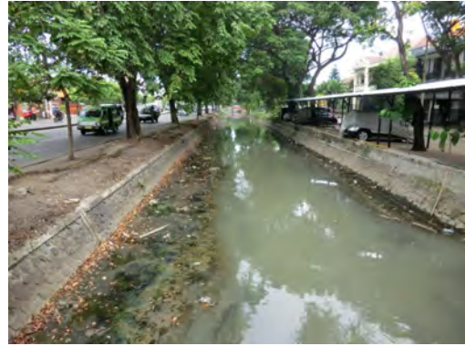
Photo 2 Drainage: Kubong Agung Canal
