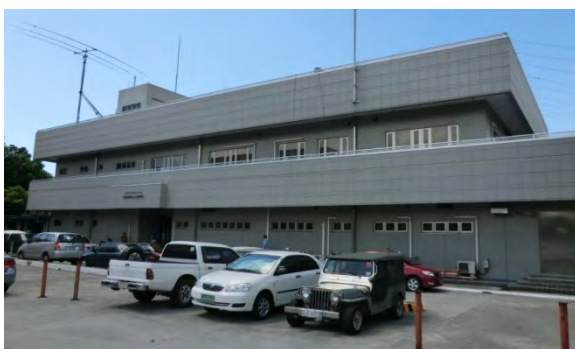
Photo 3 Manila Maintenance Center
