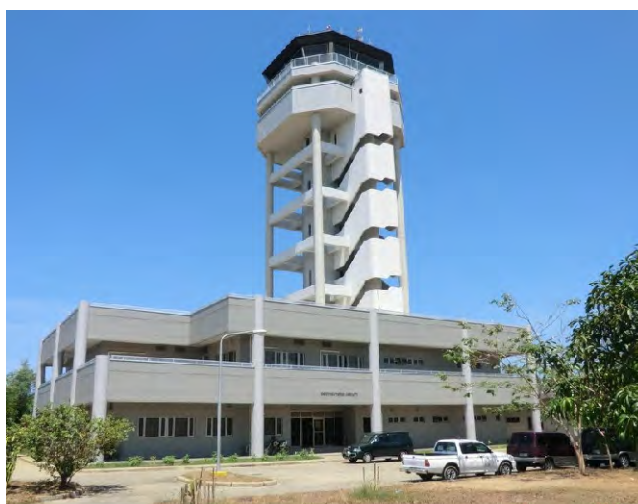
Laoag Control Tower
