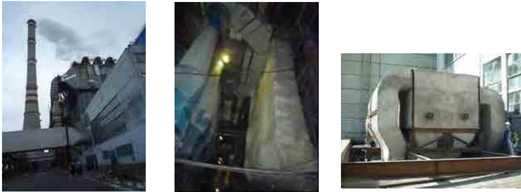
Fig. 3-5 EP (PP4), Cyclone / Venturi Scrubber (PP3, PP2)
