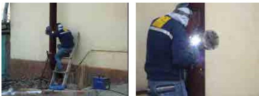
Welding sampling hole equipment (using arc welding for cast iron flue)
