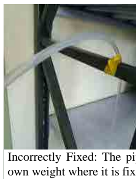
Fig. 8-4 How to Fix the Pipe
