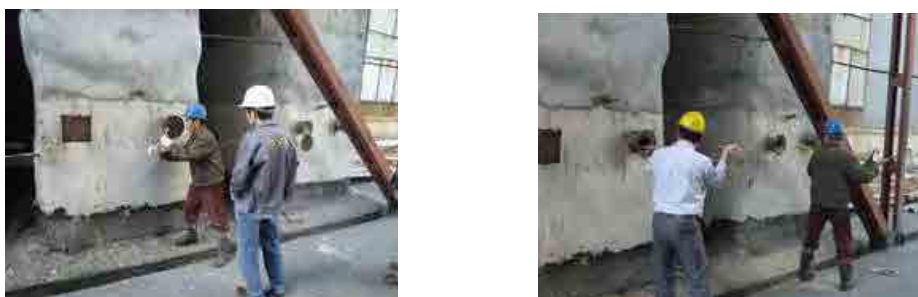
Fig. 8-19 Opening of the Measurement Hole and Cleaning Thereof
