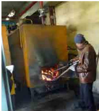
Figure 3-1 Feeding Coals into Furnace
