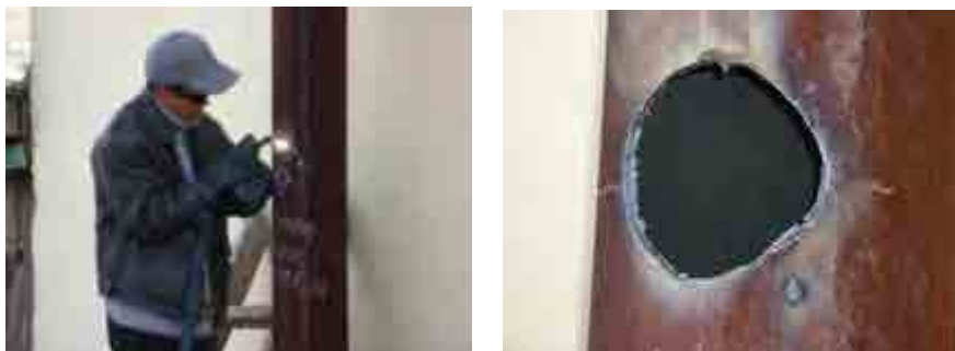
Opening a hole (using arc cutter for cast iron flue)
