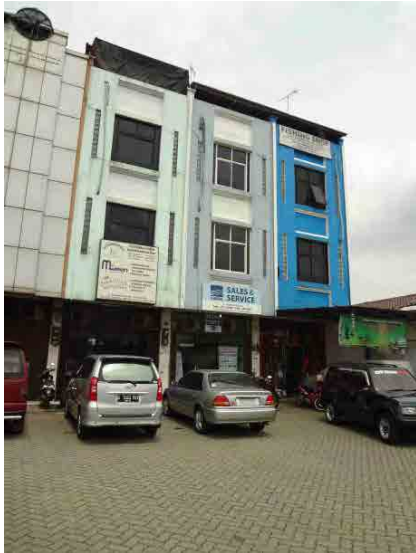
▲ Building of PT. Minori (light green one)
