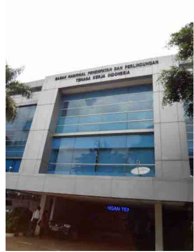
▲ Building of BNP2TKI
