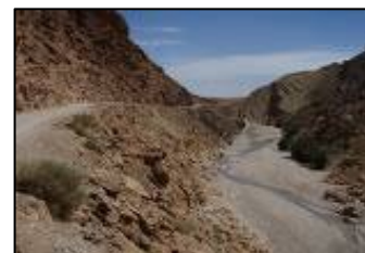
Timkid Dam Site to be scheduled the construction in Oct. 2009
