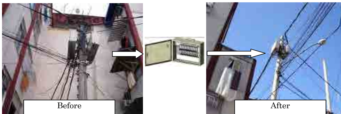
Fig. 3.3.10 Before and after of Distribution Lines to Consumers
