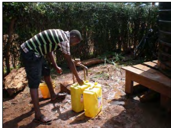
Water tap installed at individual house. Volume of water is recorded by the indicator
