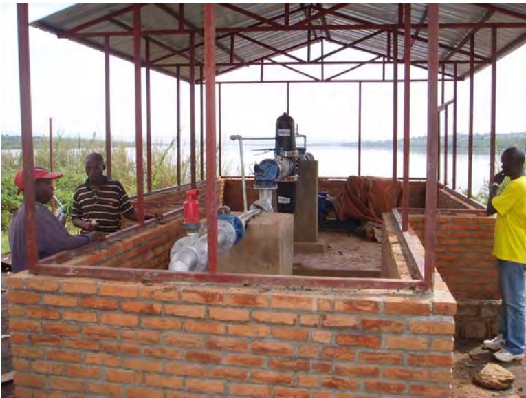
Pump station under construction by assistance of Luxemburg.
