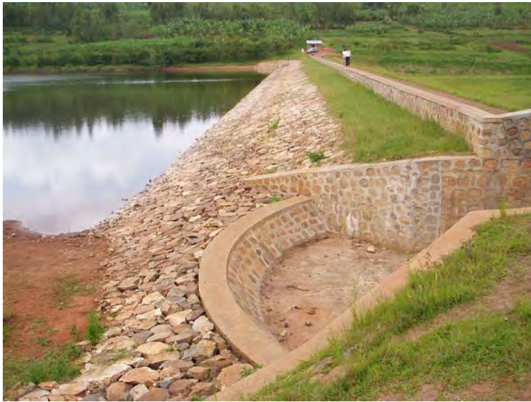
Kanyanyanba Dam. Constructed by RSSP Project.
