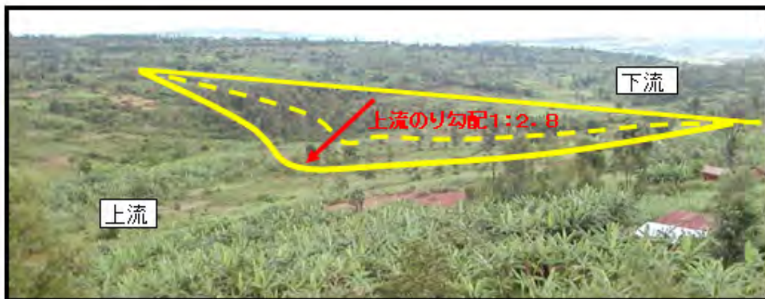
Figure 2.1.51 Image of completed dam body
