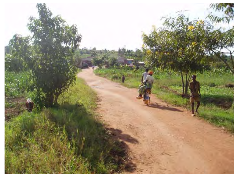
Bugesera2 Village road at downstream. The left side is upstream side. There is no drain canal. The road is overflowed a few times a year. There is Lake Rumira about 200m in the right side.
