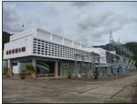
Photo 1: Da Nhim Power Station
