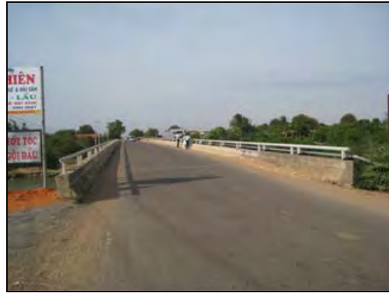
Photo 7: Luy river bridge
