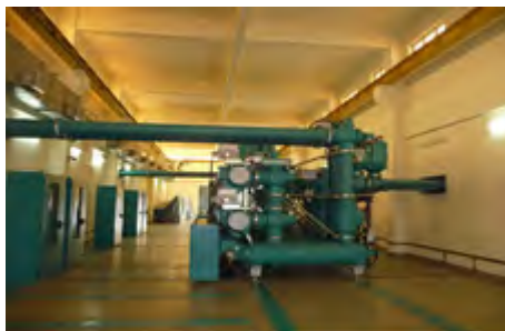
Islamabad University Substation, Bus Bar
