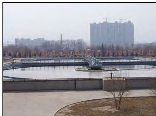
Sewage treatment plant (final settling tank)
