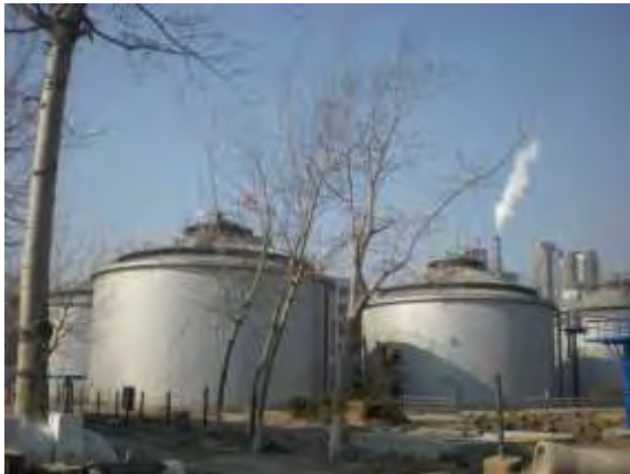
Fig. 13 Sludge digester chamber 35 (Jizhuangzi Sewage Treatment Plant)
