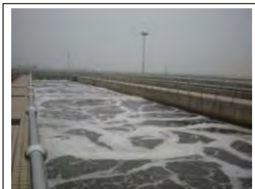
Shaoxing Sewage Treatment Plant
