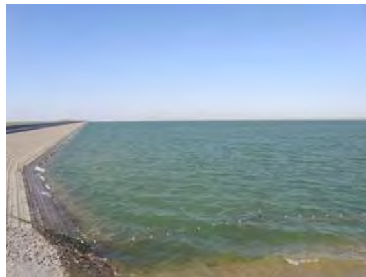
Fig. 11 Water Reservoir in Daluhu Area
