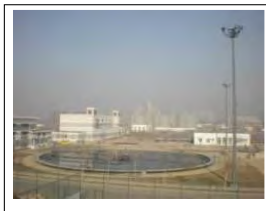
Xianyanglu Sewage Treatment Plant
