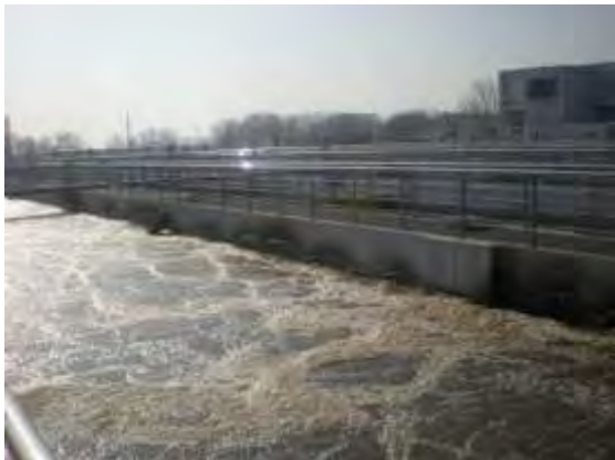
Fig. 2 Jizhuangzi Sewage Treatment Plant aeration tank
