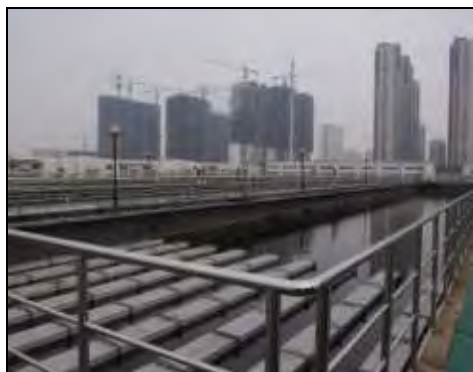
Fuxin Treatment Plant
