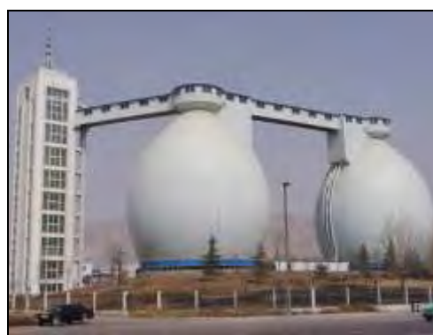
Fig. 13 Sludge Processing Facilities
