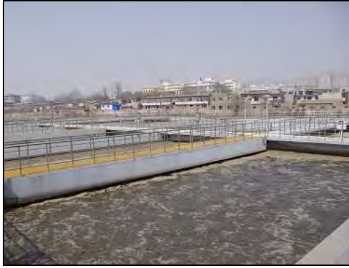
Fig.2 Biological Treatment Basin at the Sewage Treatment Plant
