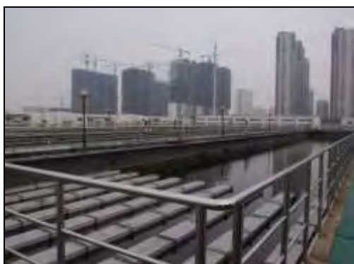
Fig. 4 Biological Reaction Pond, Fuxing Plant
