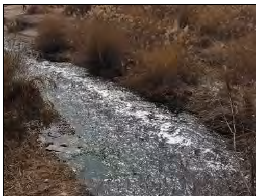
Fig.8 Discharge Outlet for Treated Sewage
