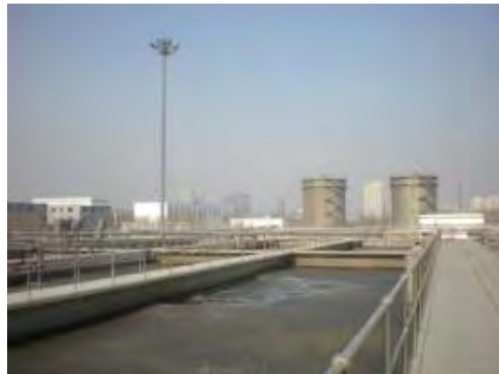
Fig. 3 Xianyanglu Sewage Treatment Plant aeration tank
