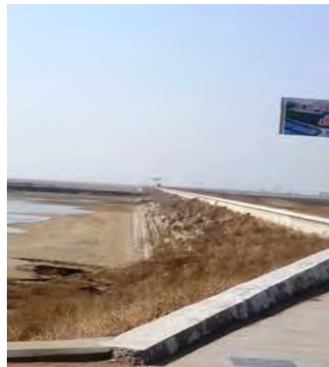
Fig.5 Embankment in the Xiazhen area
