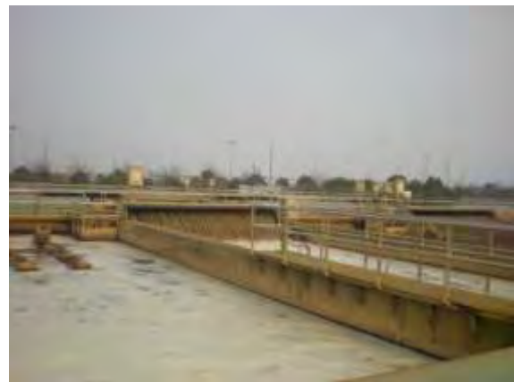
Fig. 3 Oxidation ditch (Jiaxing Sewage Treatment Plant)
