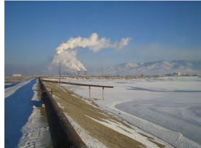
(TPP4, View from the Ash Pond)
