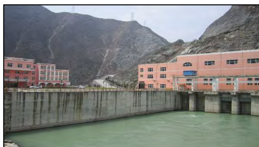
(Turbine Building, Hepingzui Hydropower Plant)
