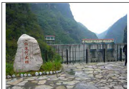
Changyang Zhailaihe Hydropower Plant
