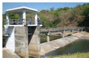
Intake weir constructed in the project
