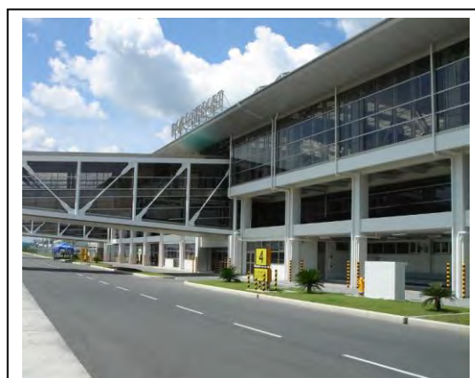
New Iloilo airport (Passenger Terminal)
