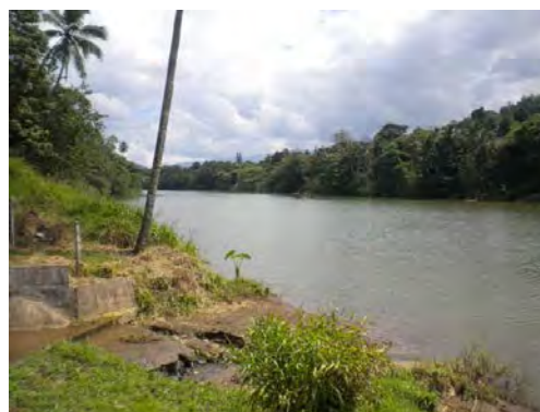
Getambe Water Intake Point (This Project)
