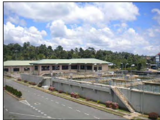
Katugastota Water Treatment Plant
