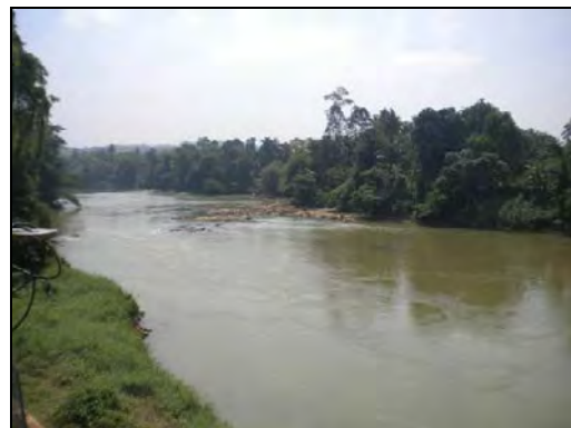
Water Intake Point of the Treatment Plant
