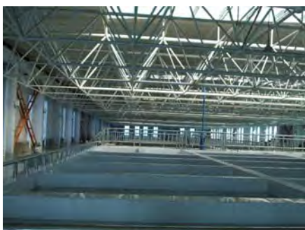
Wafangdian Water Treatment Plant
