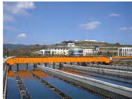
No. 7 Purification Plant (Sedimentation Pond and Office Buildings)
