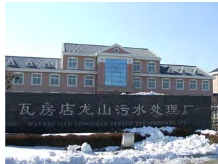
Wafangdian Wastewater Treatment Plant
