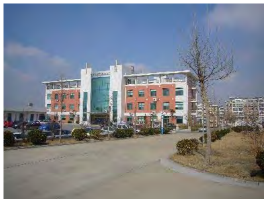
Purification Plant in Zhaoyuan (Office Building)
