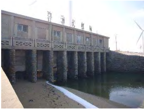
Water Gate in Laizhou (New Construction)
