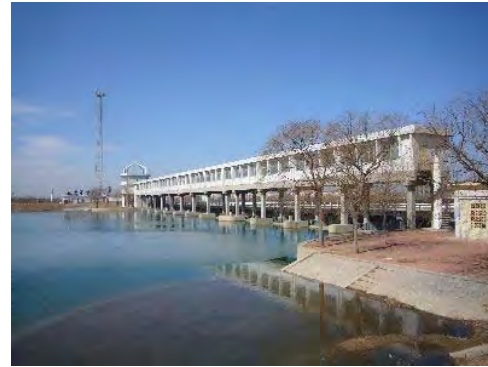
Underground Dam in Laizhou (New Construction)
