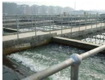
Plant C, Chengdu Sixth Water Purification Plant
