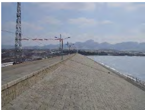
Wangwu Dam in Longkou (Rehabilitation Work)
