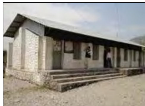
Classroom Constructed in the Project (Makawanpur District)
