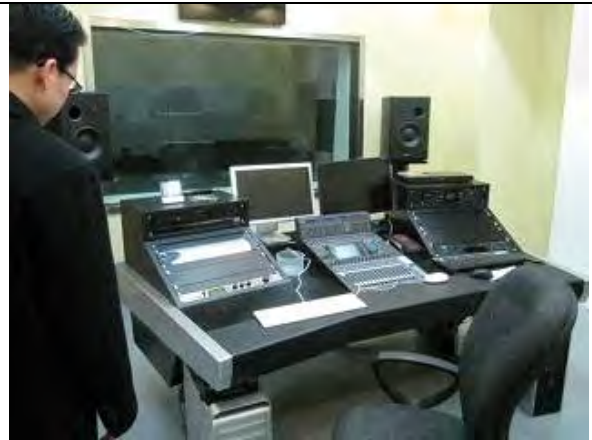
Photograph 2 Newly installed equipment (RL)
