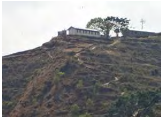
Photo 5: Classrooms Constructed by the Project on the Hilltop
