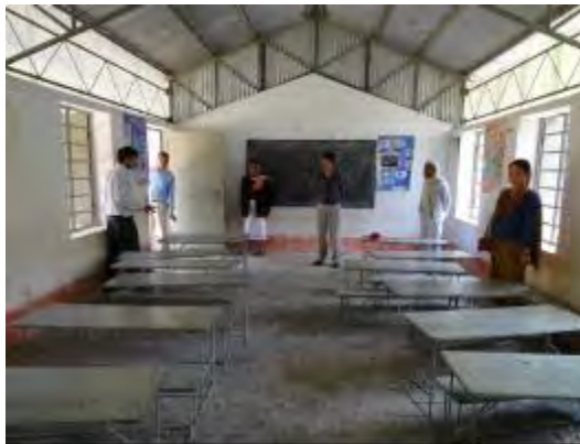
Photo 1: Interior of a classroom constructed with community participation in this project
