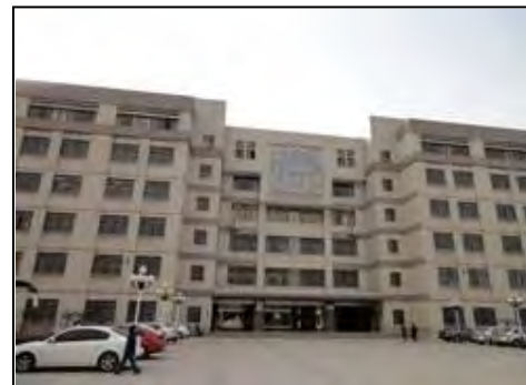
University Building Constructed by the Project (Xi’an University of Technology)
