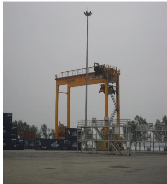
Cranes installed at Cai Lan Port
