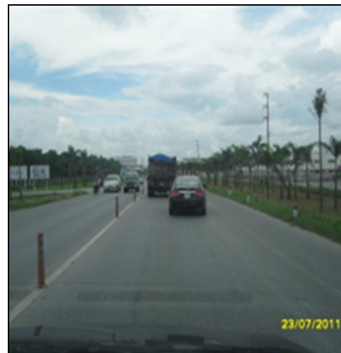
National Highway No. 18
