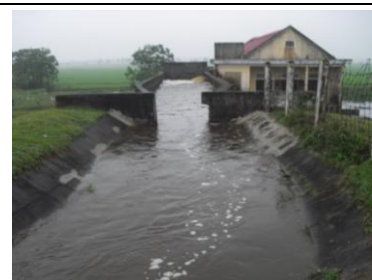
The rehabilitated irrigation
