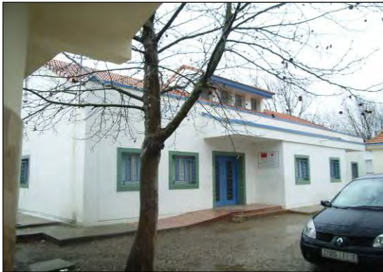
Picture 1: Immouzer Urban Health Center with a Maternity Unit constructed by the Japanese Grant Aid Phase I. (Séfrou Province)
