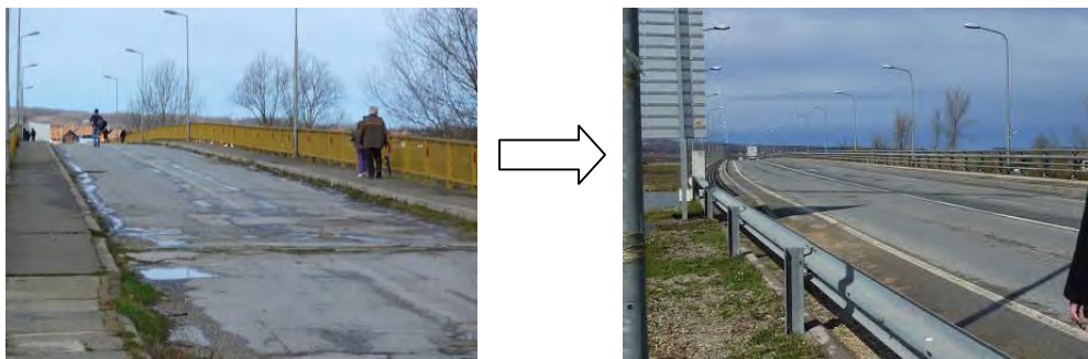
Figure 3: Change Before and After the Project Implementation (Modrica Bridge)
