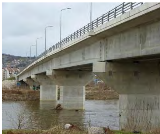
New Doboj Bridge
