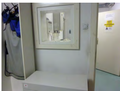
Figure 2: Renovated Monitor Window and X-ray Sealed Door (X-ray Room) (Banja Luka, RS)
