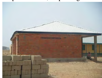
Photo: Classroom constructed by a SUBEB (Kaduna) by adopting JICA's design
