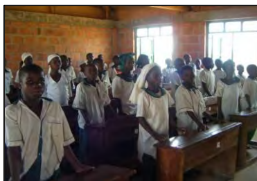
Photo (left): A classroom where chairs and desks have not been installed (classrooms in such circumstances are still common in Nigeria today)
