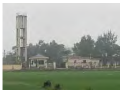
Water Plant in Van Thang, Thanh Hoa
