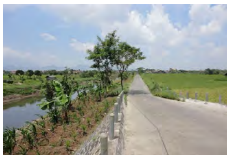
Access road constructed under the project
