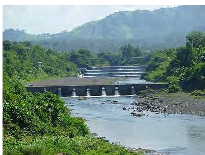
Figure 20: Sand-control Dam in Bali's Largest River (Unda River)
