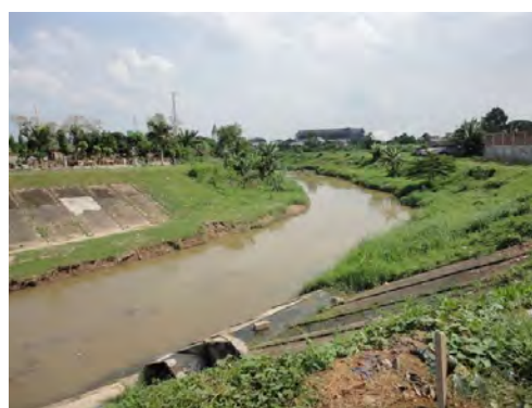
Percut River after improvement
