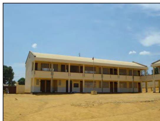
External appearance of a constructed school building (Primary School of Ebolowa in South region)
