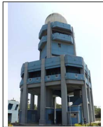
Khepupara Radar Station
