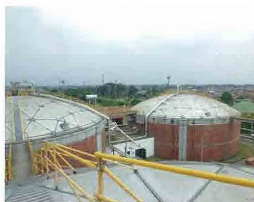
Overview of the sewage treatment plant
