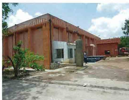
Water supply facility in Hyderabad
