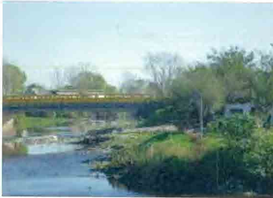
Photo 5 The Taurita Bridge
