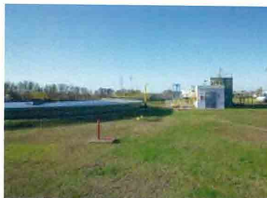
Photo 4 San Miguel Disposal Plant
