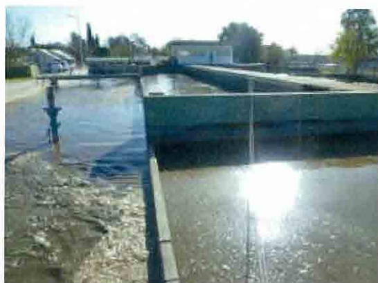
Photo 3 Hurlingham Disposal Plant
