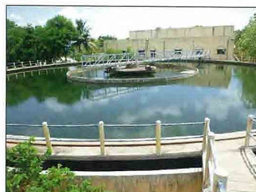
Filtration Plant in Hyderabad
