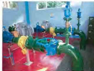
Upgraded equipment in facilities Bolabog Pumping Station
