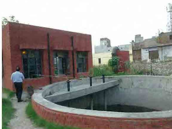
Sewerage facility in Amritsar
