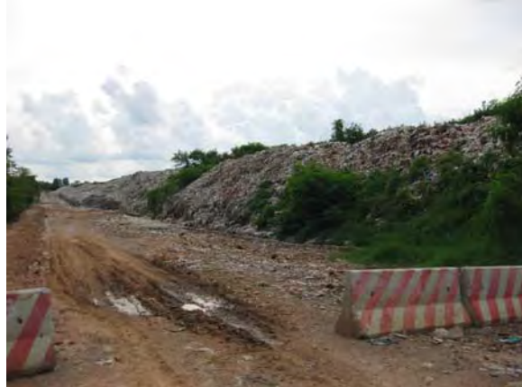
Sanitary Landfill in Khon Kaen
