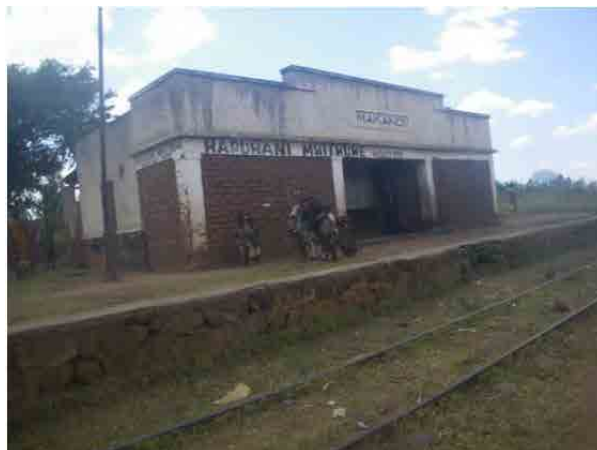
Photo A5-15 Makande Station
