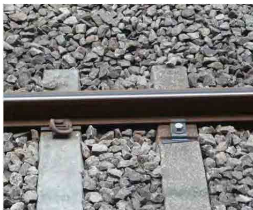
Figure 9-26 Fastening System (Double Elastic Fastening and Clip-type Fastening)
