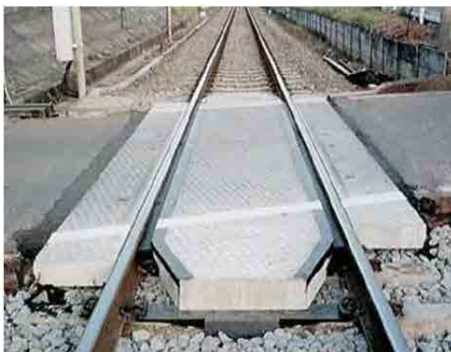
Photo 9-4 Example of Crossing with Precast Crossing Plate
