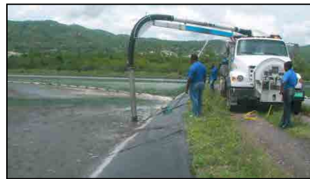
Photo 16 Cleaning of Wastewater Stabilization Pond
