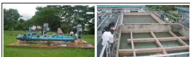
Photo 3 Logwood Water Purification Plant
