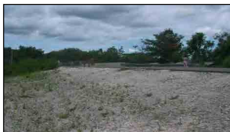
Photo 18 Road after Reinforcement
