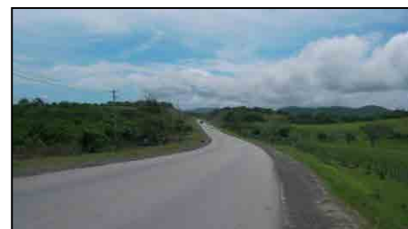
Photo 6 General Condition of Road
