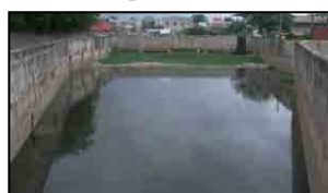
Flood Drainage Facility
