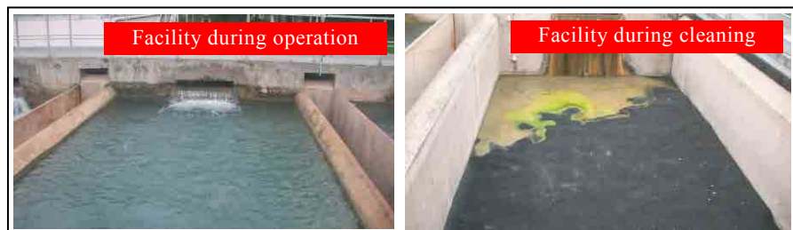
Photo 15 Maintenance of Water Supply Facility
