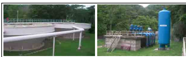
Photo 4 Great River Water Purification Plant
