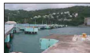
Pier at Ocho Rios Port
