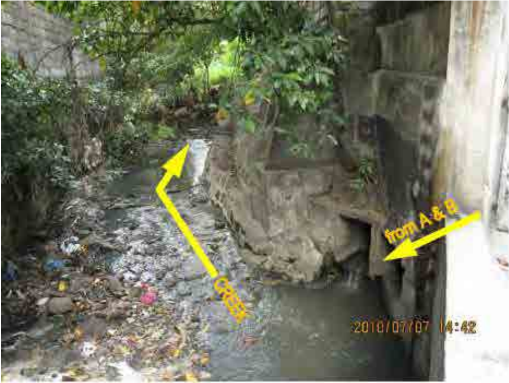
Picture. 5-5 Detail of the Creek Discharging Mouth (Parañaque)
