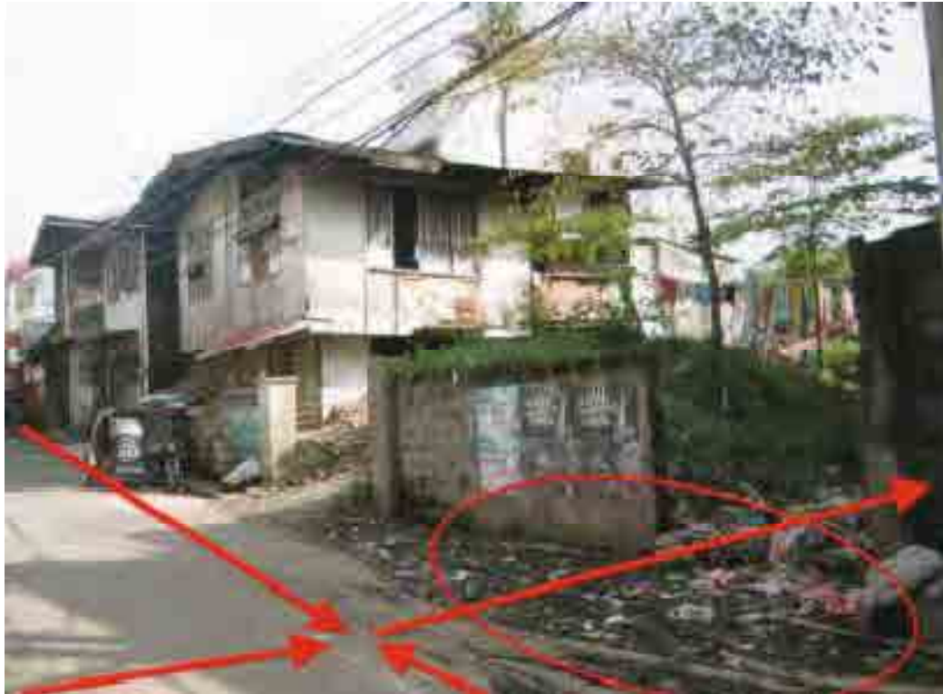
Picture. 5-7 Garbage Accumulated at the Creek Discharging Culvert
