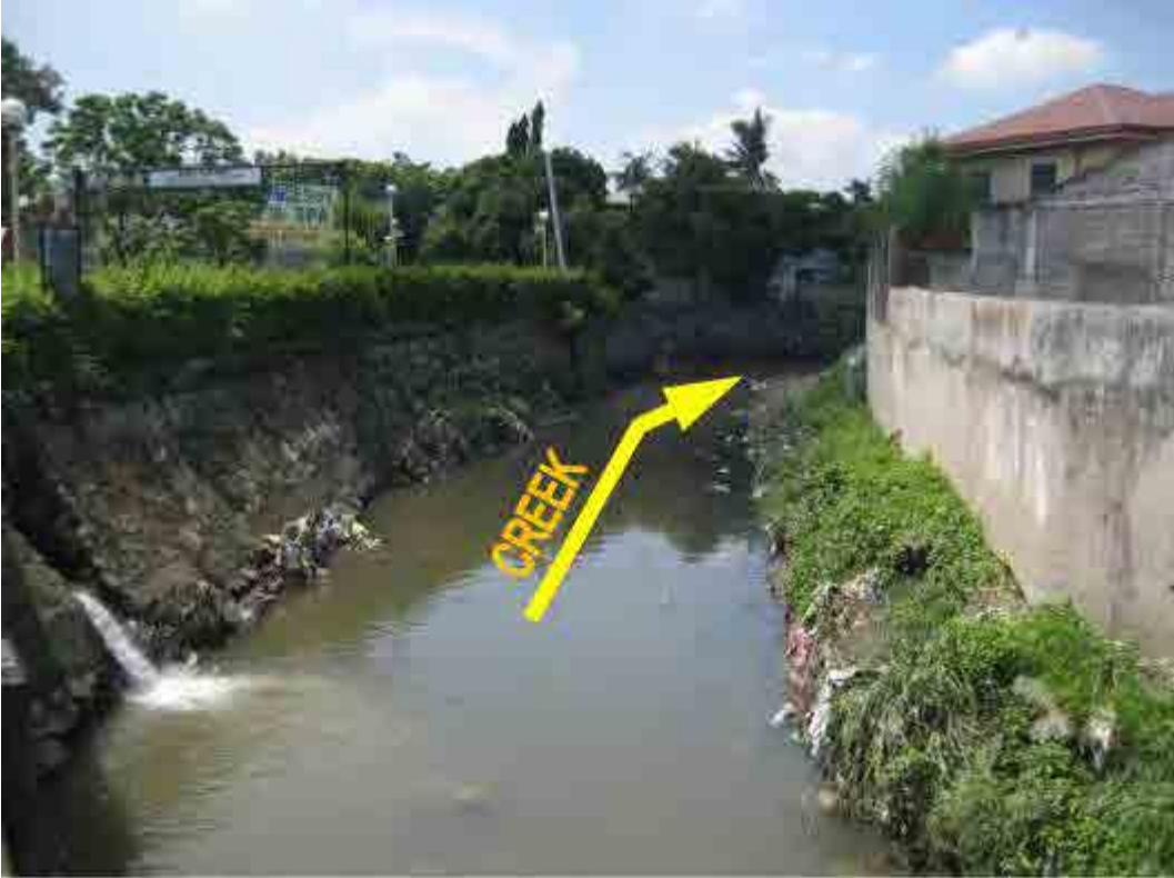
Picture. 5-6 Another Creek (bigger) Meeting Point to the River (Las Piñas)
