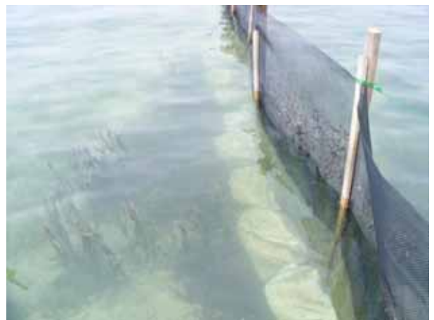
Sand bags to hinder spats escaping and strengthening the pen at Mandathivu
