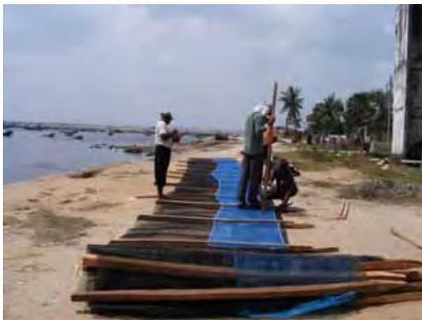
Pen construction in progress at Gurunagar
