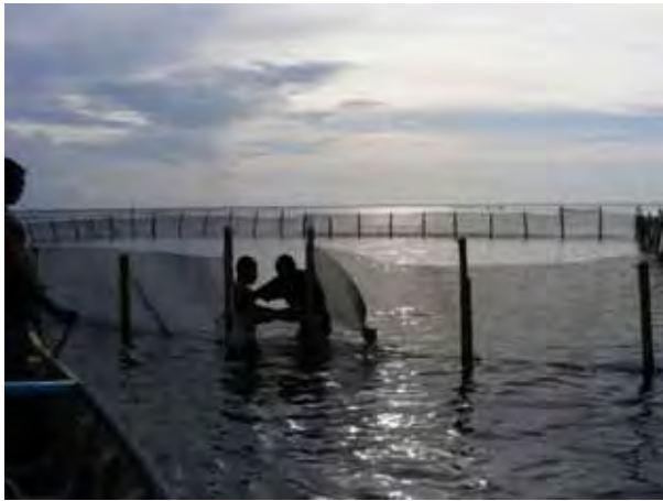
Pen construction in progress at Navanthurai
