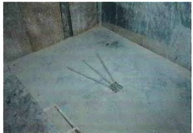
To guide juice from silage to the catch basin, three ditches were provided
