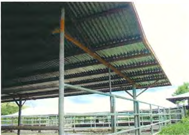
Extended roofing from the low angle
