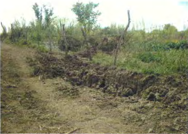
Actually, this is a puddle, one of the heavy damaged portions on the road
