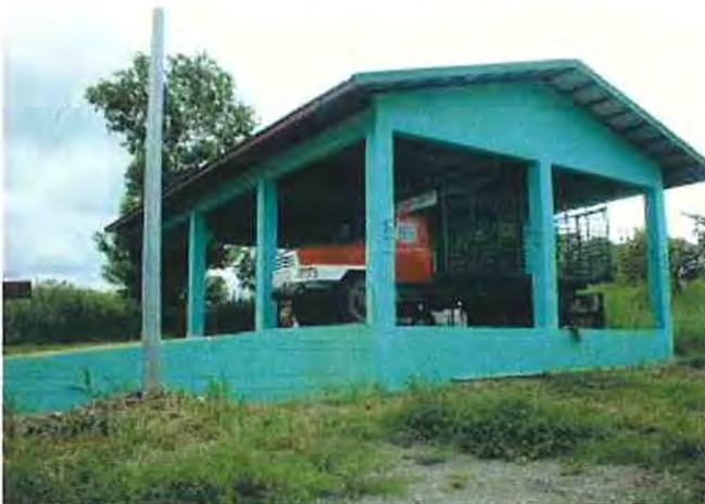
The rest area has enough space for parking a big truck
