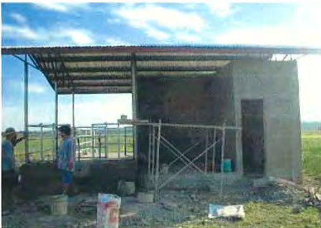
An overall view (under construction)
