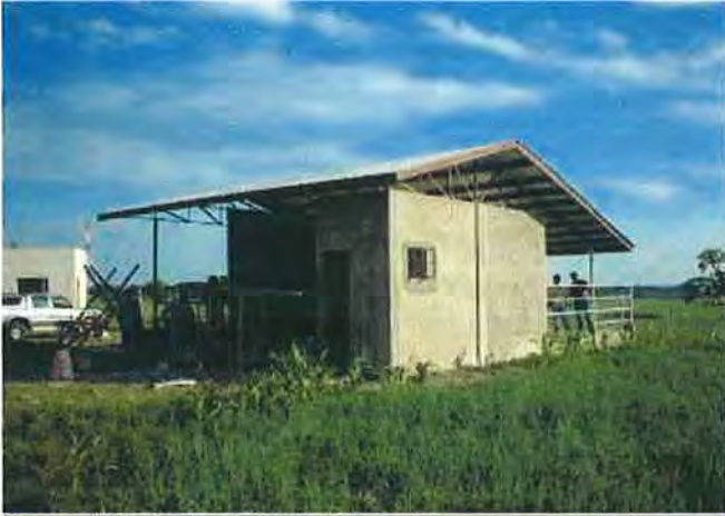
An overall view (under construction)
