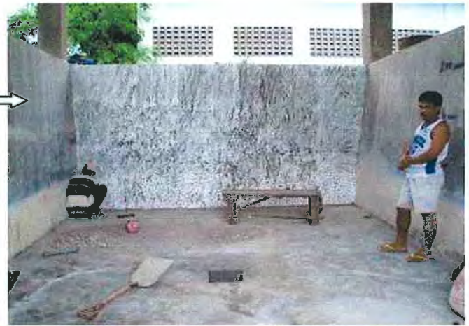
Chipping of damaged portion before plastering
