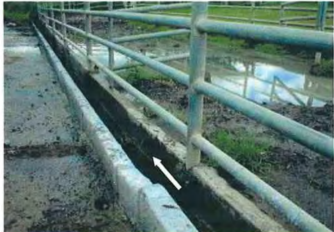
Leading mud and rain water to the indicated direction to drain
