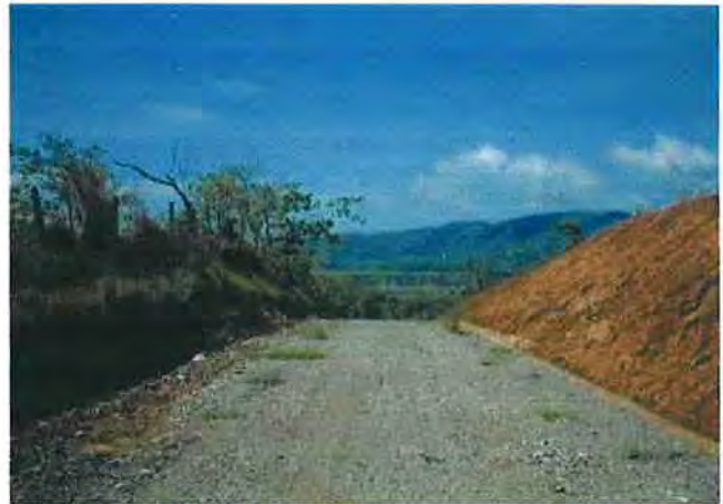
Adjusted slope and smooth road surface
