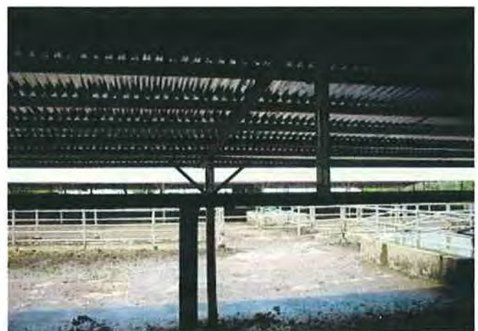
Extended roofing from the low angle
