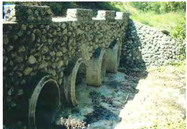
A view of upper stream where the barrels installed
