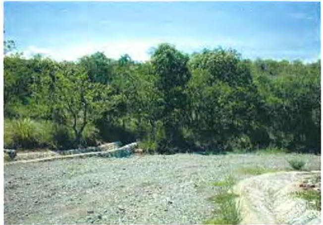
Rip rap canals were installed on both sides
