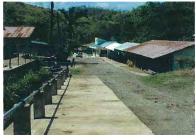
A view of location of exercise railings, bull shed and laboratory facilities (white roofing)
