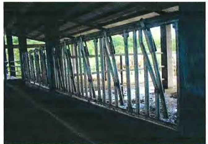
Two sets of stanchion are installed for each pen
