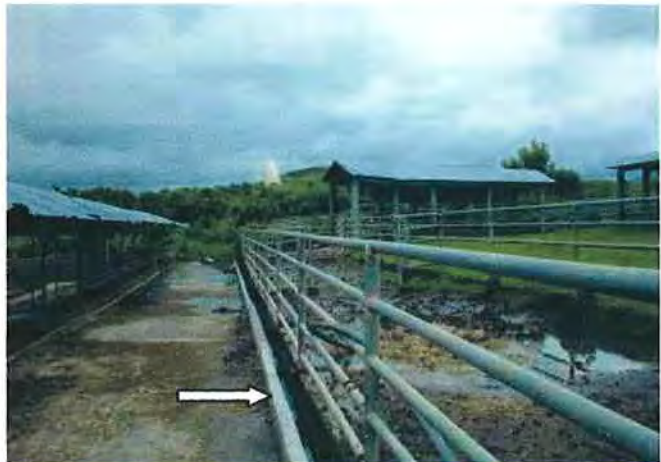
Receiving and draining mud and rain water from gate way to the weighing area
