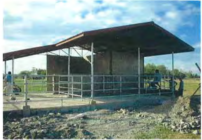
An overall view (under construction)
