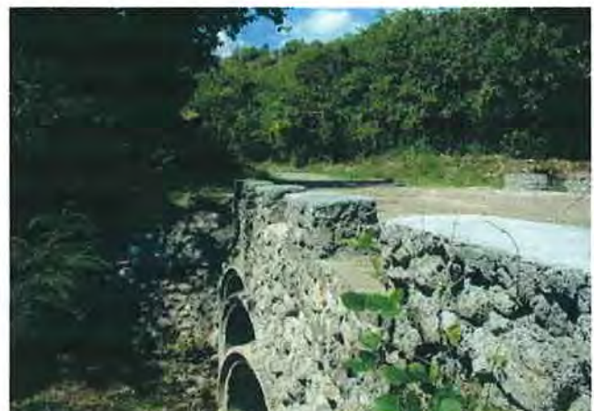
A view of down stream where the barrels installed
