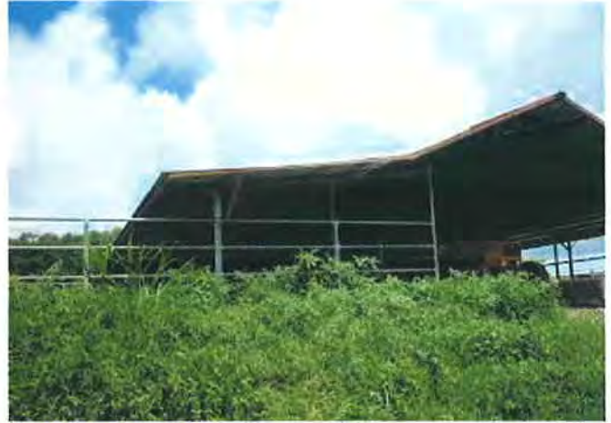
A side view of extended roofing
