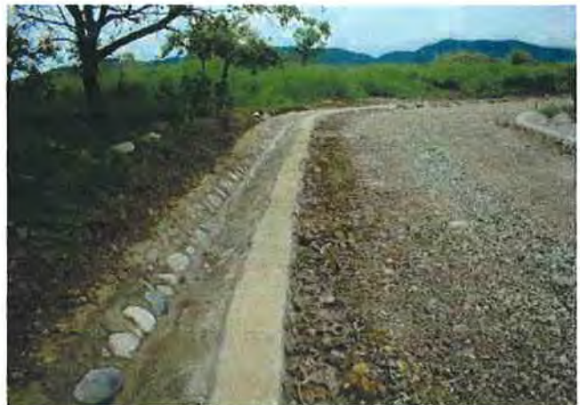
A rip rap canal was also installed
