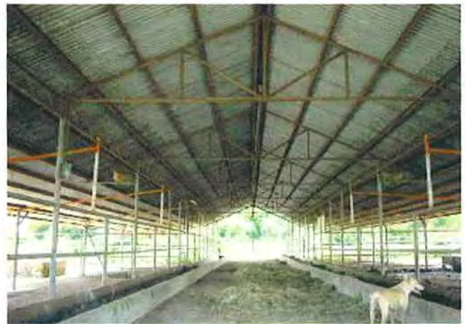
A wide view of roofing from the low angle
