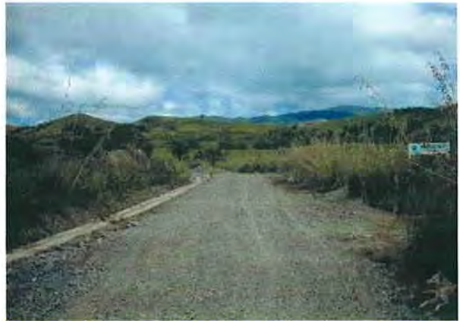
Rehabilitated road condition with a rip rap canal
