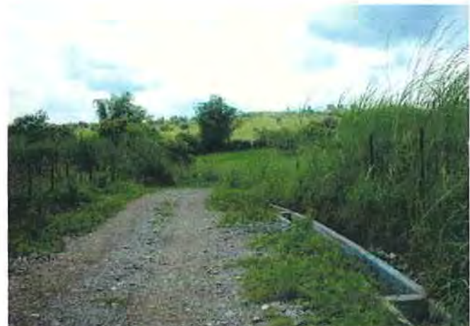
A box-drainage was established along the road
