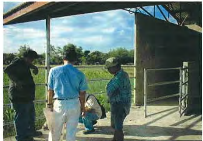
Reconfirming a location of the watering and feeding troughs (under construction)
