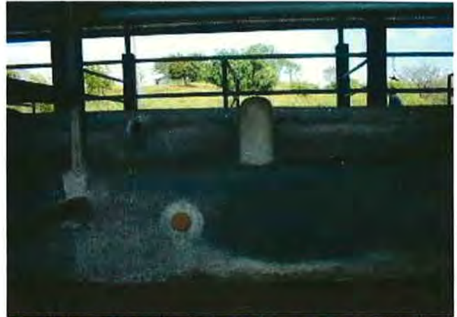
A big size of drain (red color cover) for each watering trough is installed
