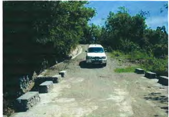
A view of road condition over the barrels with concreted surface
