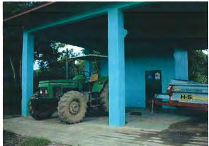
Enough spaces for tractor (left) and manure spreader (right)
