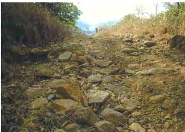
So many big stones were buried
