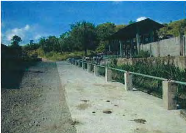
Cemented floor with concrete poles and steel pipes for railing
