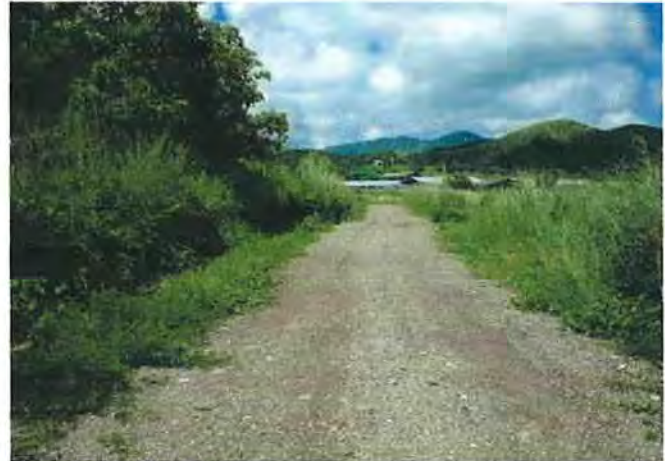
Gravelling with compaction
