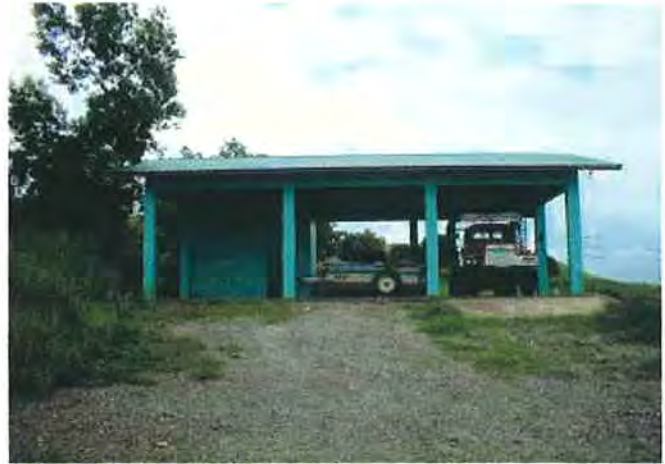
A front view (It is divided by three areas)
