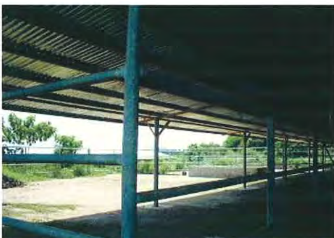
Extended roofing from the low angle
