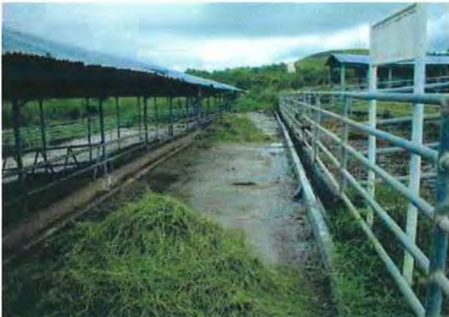
This drain system also keeps the working corral in between calf pen and gate way clean
