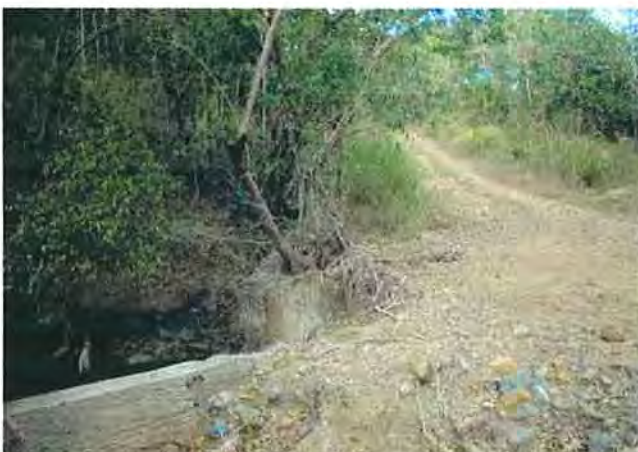
A view of down stream where the box culvert located
