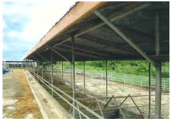
Re-welded railings
