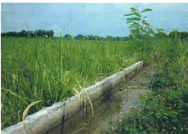
A rehabilitated canal
