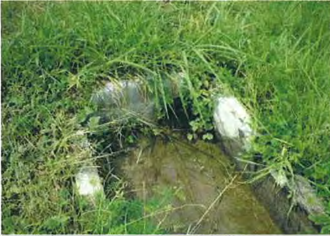
A rehabilitated gate of irrigation canal for pastureland No. 2
