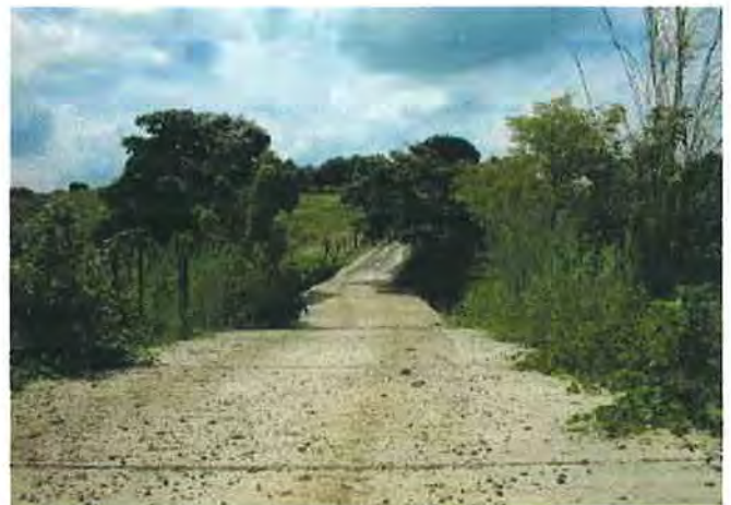
Slope was concreted with steel bars inside
