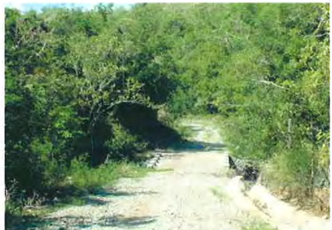
Road was filled with soil and graveled
