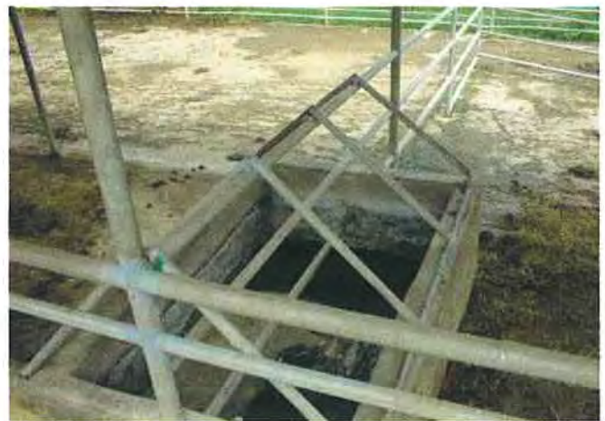
Re-welded railings
