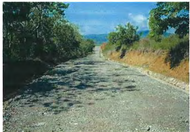
Very nice road condition
