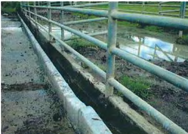
A condition of after raining
