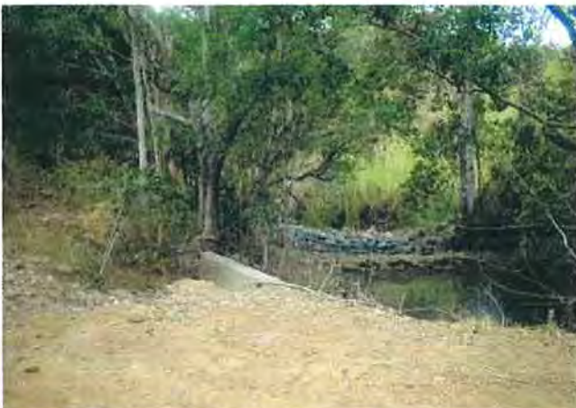
A view of upper stream where the box culvert located
