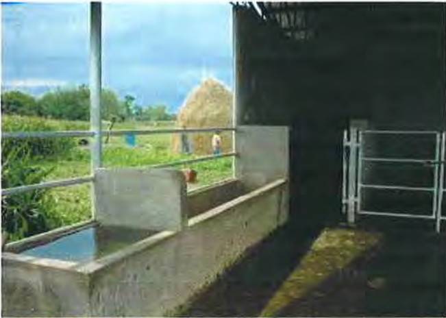
Watering and feeding troughs (completion)
