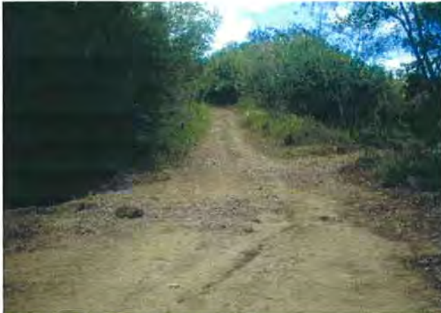
A view of road condition over the box culvert
