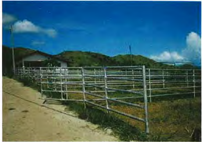
Pipes for main poles are using a size of "2" G.I.
