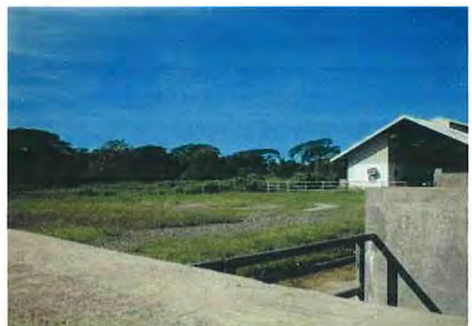
Fencing for the area of Heifer
