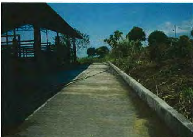
Working corral for waste management area is widen and re-cemented with edge wing
