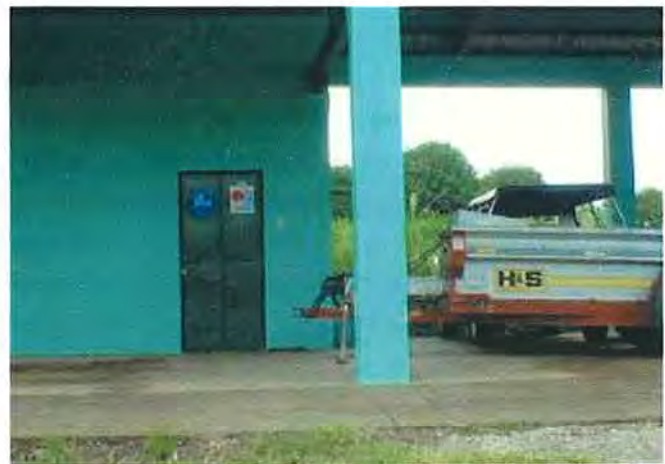
A tool room is also provided in and its door with JICA and ODA stickers
