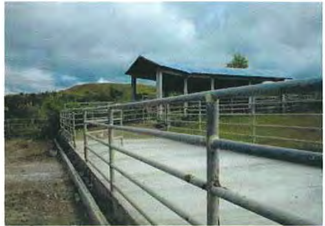
15 cm-depth concreting was executed
