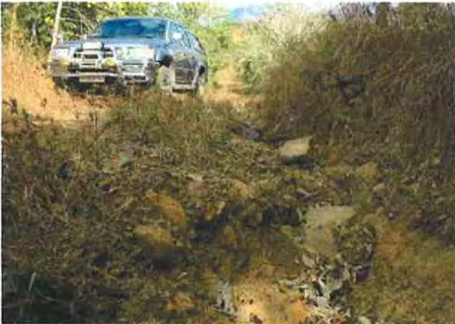
An eroded portion on the shoulder
