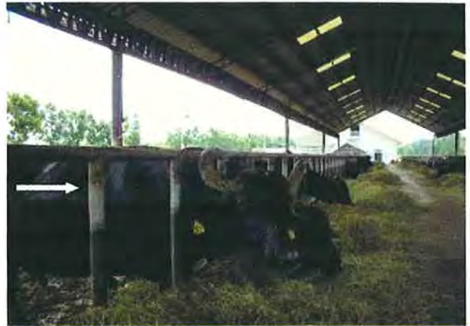
Pipes painted gray color were added
