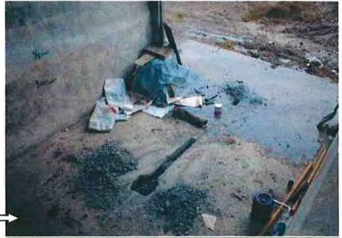
Ditch making for drain pipe
