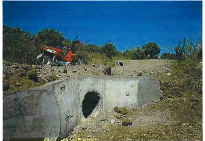
A culvert was installed to drain water
