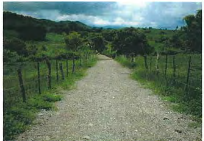
Also slope was concreted with steel bars and continuous graveled road
