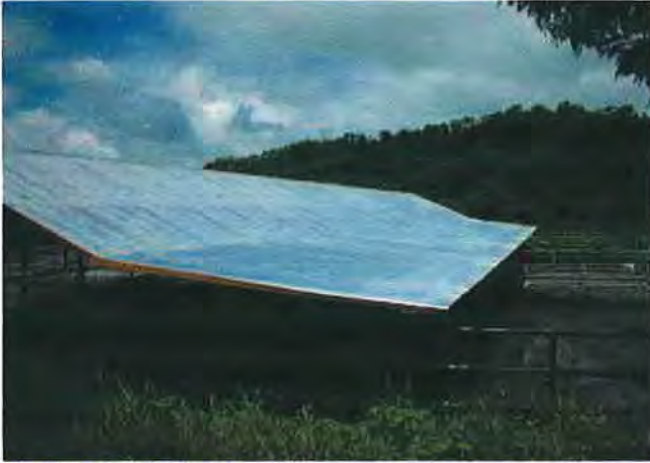
An overall view of extended roofing
